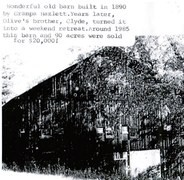
The old barn from the road below located near Georgeville which is 20 mi. south of Punxsutawney, PA
